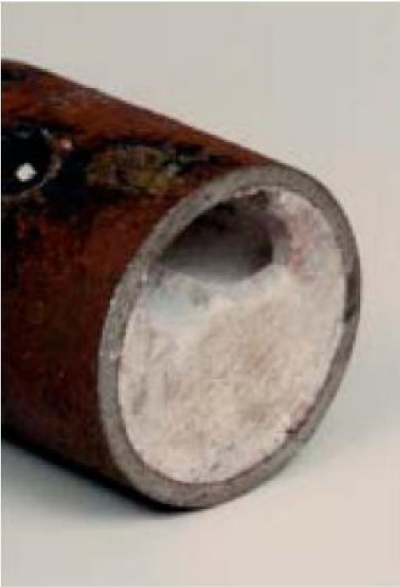
Boiler scale on water side
