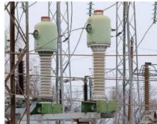
SF 6 110 kV current transformer TGFM series, Russia
