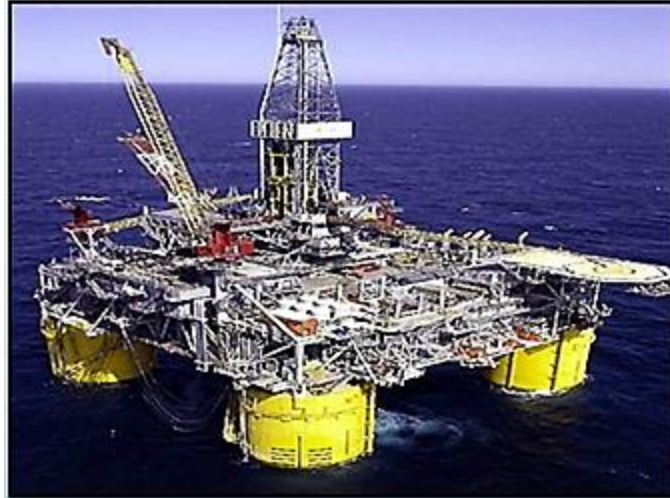
Figure (4), Positioning of Huge Offshore Platform
